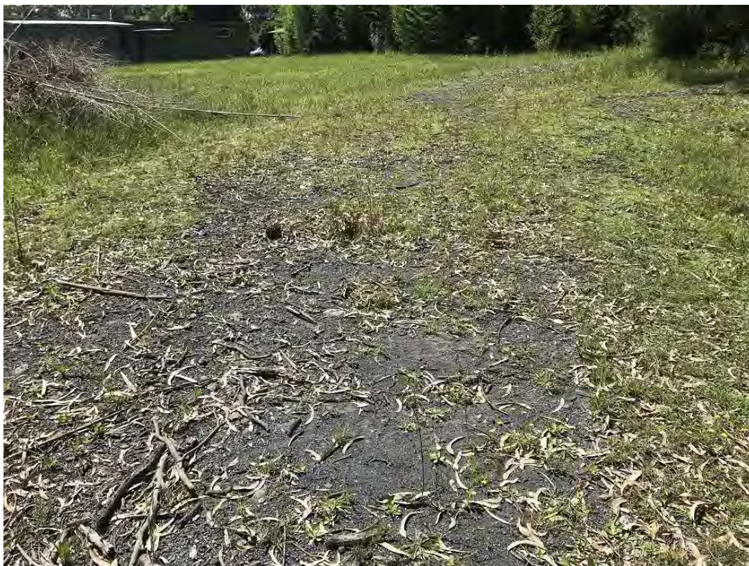
Plate 15 – Imported gravel material used for access road on Lot 11 DP 777034. Sample location TP19. Date: 14/01/2021
