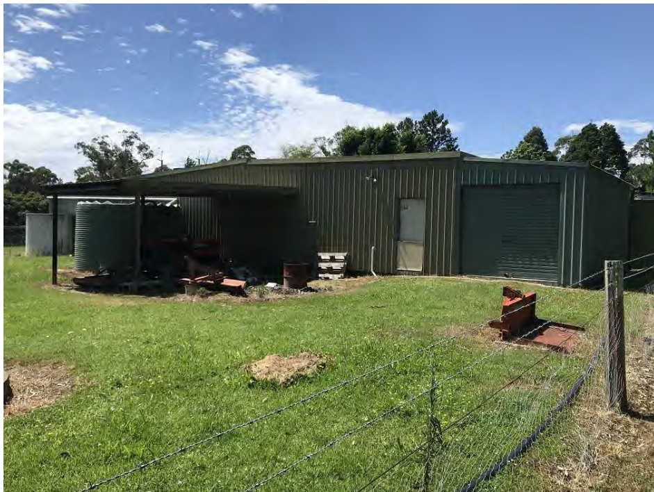
Plate 18 – Rear of dwelling on Lot 2 DP 529914. Date: 14/01/2021
